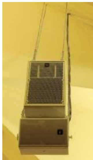
Hakka Methodist church is now served by L-R arrays comprising KV2 ES1.0 speakers with ESD10 downfills
