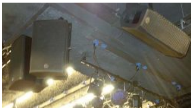
Clair Brothers R2D-64 speakers deployed at FOH and combined with F-28 side fills
